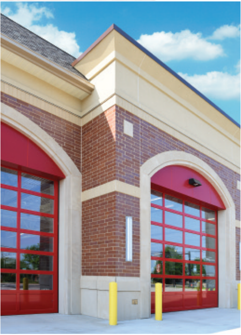
Each of the apparatus bays features a two-piece cast stone system surrounding the 14-foot high arch with cast stone affixed to premade lintels.
