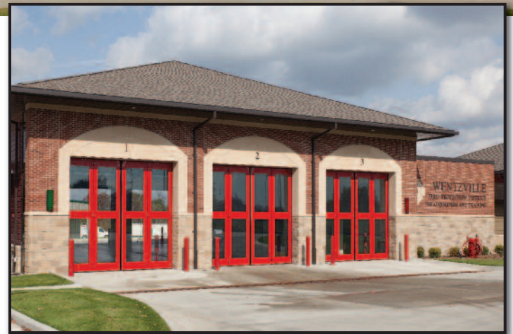
The apparatus bays display the beautiful combination of brick, cultured stone wainscoting and cast stone arches.
