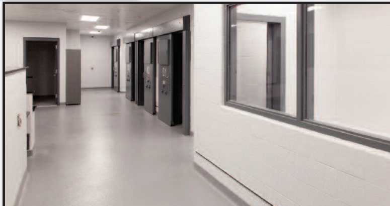
The highest security areas of the building are constructed of CMU for security, durability, low maintenance and acoustics.
