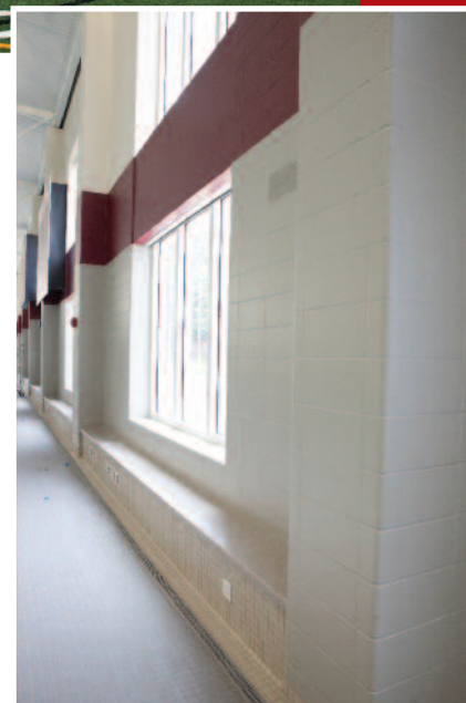
THE INTERIOR OF THE AQUATIC CENTER IS A "MOIST BOX". BEHIND THESE BLOCK WALLS IS A CAVITY DRAINAGE SYSTEM FOR POTENTIAL CONDENSATION.
