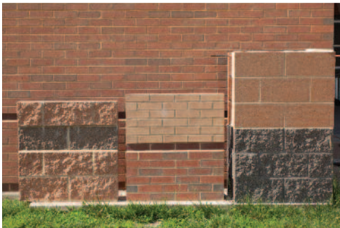
THESE TEST WALLS SHOW THE DIFFERENT TREATMENTS OF BRICK AND BLOCK USED ON THE NEW ADDITION.
