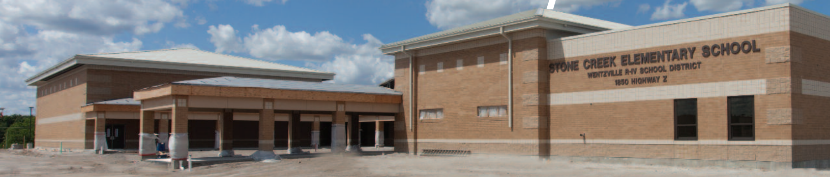
THE WENTZVILLE SCHOOL DISTRICT SELECTED A BUFF COLORED BRICK AND LIGHT BLOCK AND STONE ACCENTS FOR THEIR TWO NEW ELEMENTARY SCHOOLS – STONE CREEK AND WABASH – IN ORDER TO BEST INTEGRATE INTO THE SURROUNDING COMMUNITIES.
