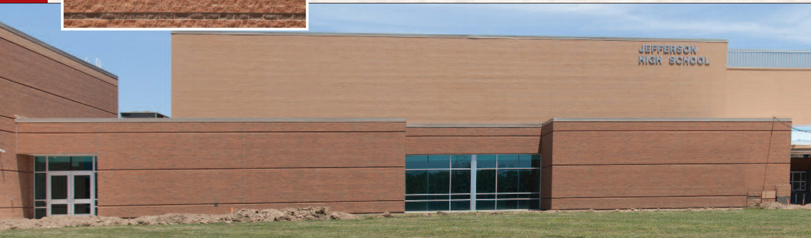
SINGLE COURSES OF CHOCOLATE BRICK BREAK UP THE SPLIT FACE CMU ON THE SIDE WALL OF THE NEW ADDITION.
