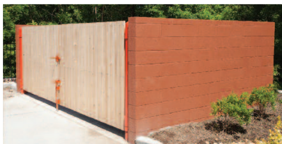
THE CMU WASTE RECEPTACLE ENCLOSURE PROVIDES EXTRA DURABILITY NEEDED FOR THE EXPECTED HEAVY USE.
