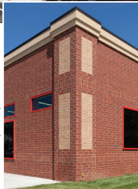
INSETS OF BUFF BRICK MASONRY HIGHLIGHT THE OFFSET PILASTERS ORNAMENTS THE BUILDING'S EXTERIOR.
