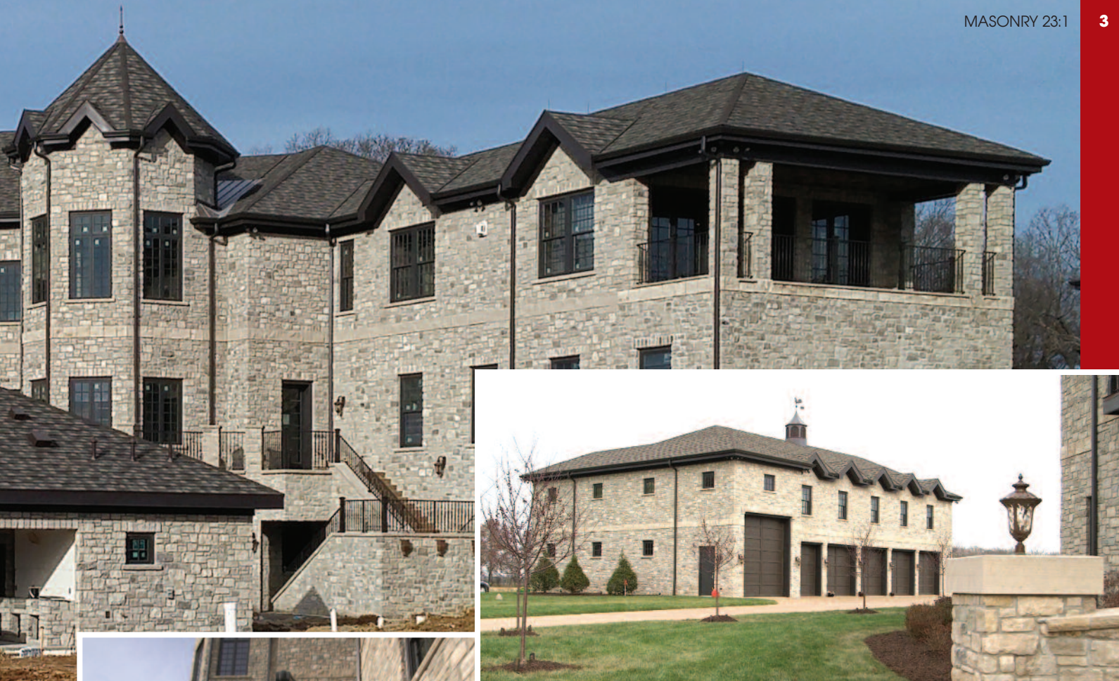
THE STONE IN THE 9,000 SQUARE FOOT CARRIAGE HOUSE MIMICS THE ASHLAR PATTERN AND SMOOTH FACE LIMESTONE BANDING BETWEEN FLOORS ON THE MANSION. PHOTO BY CREATIVE EDGE.
