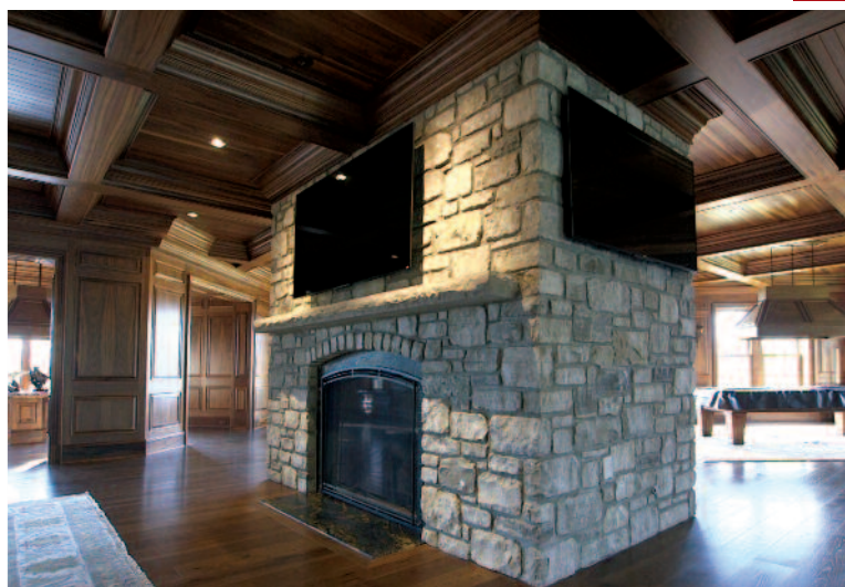
RIGHT: THE TRADITIONAL LOOK ESTABLISHED BY A THIN STONE VENEER ON ALL FOUR SIDES OF THE FIREPLACE JUXTAPOSES NICELY WITH THE LATEST IN VIDEO VIEWING ON MULTIPLE SCREENS. THE STONE MANTLE HAD CUTS MADE TO PROVIDE ELECTRICAL ACCESS. PHOTO BY CREATIVE EDGE.
