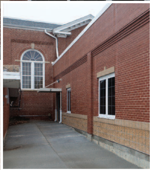
THE NEW WING TIES INTO THE EXISTING STRUCTURE IN THE CENTER OF THE PHOTO. BRICK COLOR SELECTION WAS CRITICAL TO THE SUCCESS OF THIS PROJECT.
