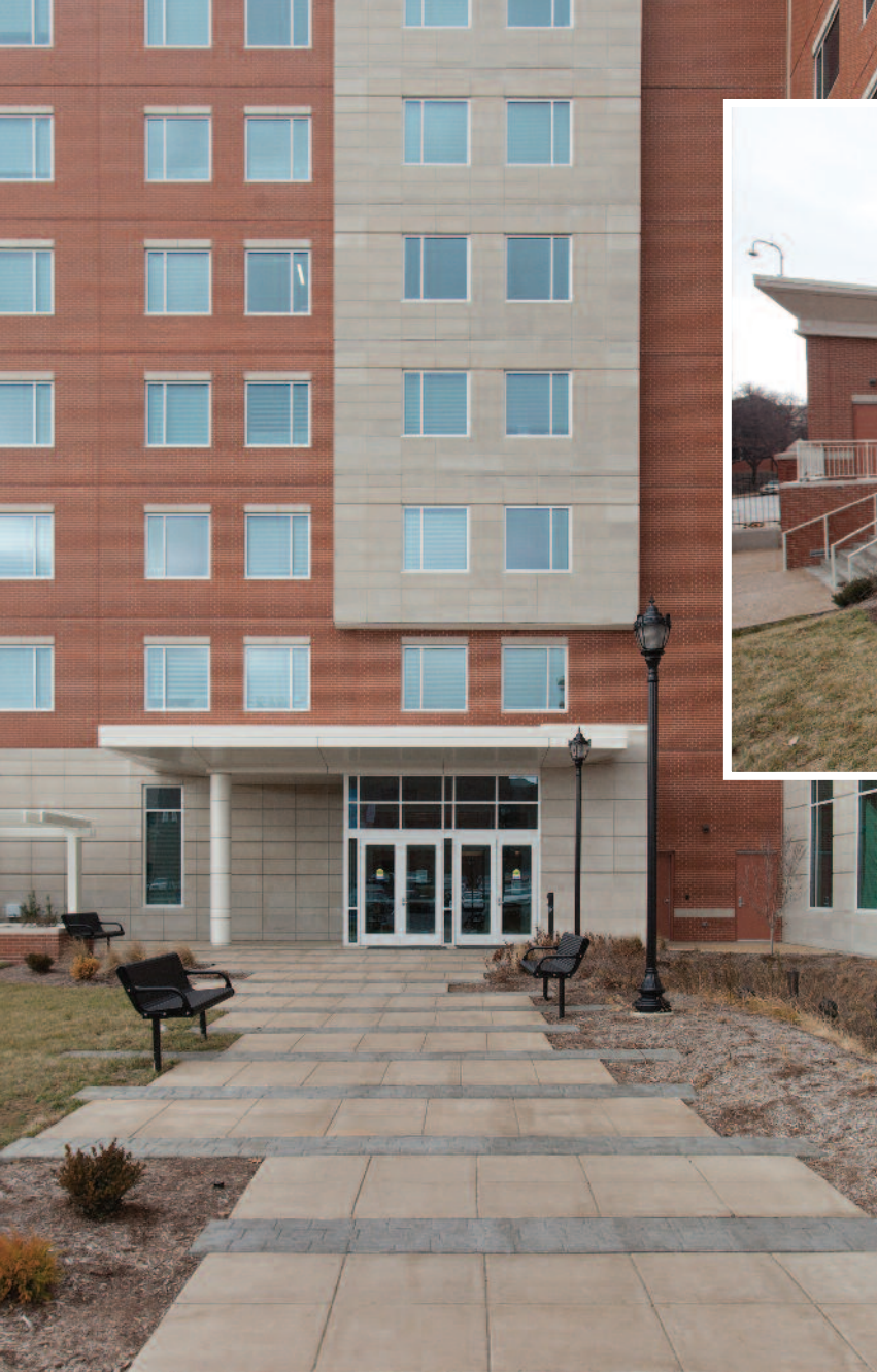
CAST STONE TRIM ABOVE THE MAIN ENTRANCE TO SPRING HALL AND A PATH OF STONE PAVERS CREATE A WARM AND WELCOMING PORTAL TO THIS NEW RESIDENCE HALL.
