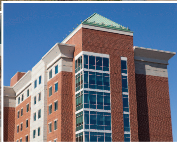
VERTICAL AND HORIZONTAL BANDS OF CAST STONE EFFECTIVELY HELP REDUCE THE MASS OF THE EIGHT STORY BRICK BUILDING.
