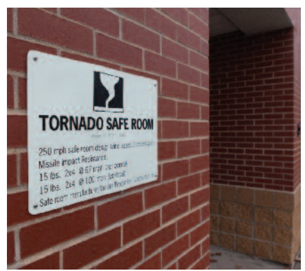
THE NEW ADDITION TO TRUMAN LEARNING CENTER FEATURES TWO SEEMINGLY IDENTICAL WINGS OF CLASSROOMS. INSIDE THE LOADBEARING WALLS OF THE EAST WING ARE THE ELEMENTS THAT CLASSIFY IT AS A FEMA RATED TORNADO SHELTER.
