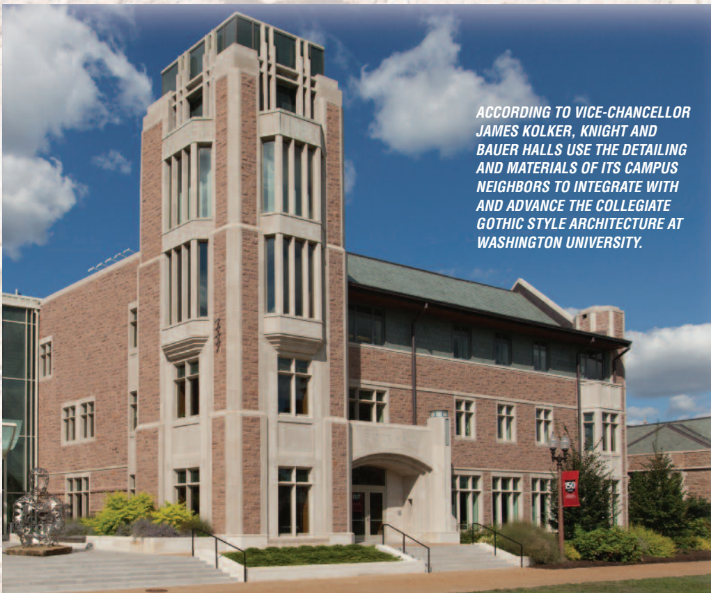
MISSOURI RED GRANITE AND INDIANA LIMESTONE AT PLAY IN A DETAIL FROM THE BAUER HALL SIDE OF THE NEWEST BUILDING IN THE OLIN SCHOOL OF BUSINESS. ACCORDING TO JOHN SMITH, PRESIDENT OF JOHN J. SMITH MASONRY, EACH PIECE OF RED MISSOURI GRANITE ON THIS BUILDING IS HAND CRAFTED IN THE MASON CONTRACTOR'S WORKSHOP.
