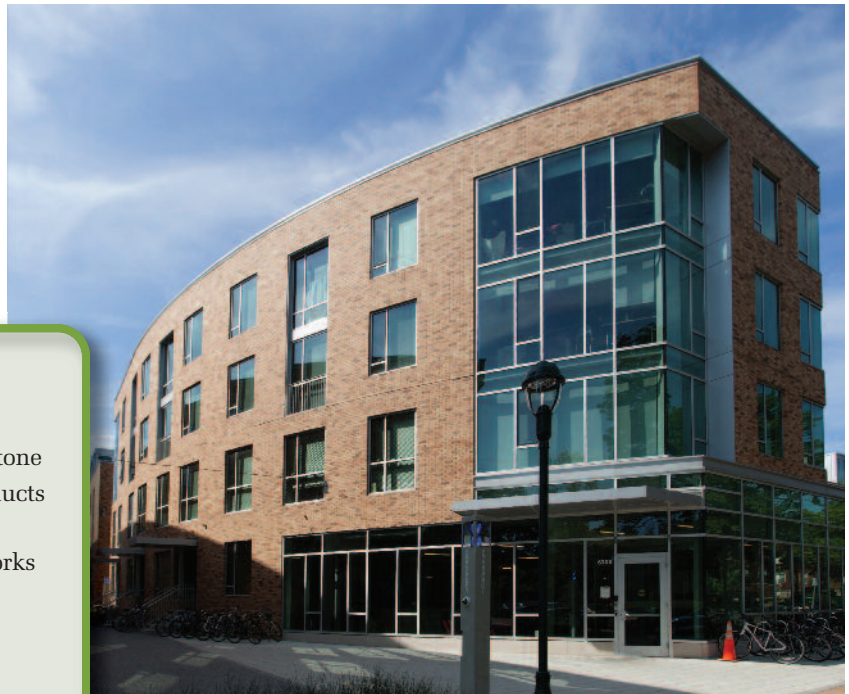
THE PEDESTRIAN MEWS LINKING ENRIGHT TO DELMAR IS FORMED BETWEEN TWO RESIDENTIAL BUILDINGS. THE CONSTRUCTION OF A RADIUS WALL ON THE BUILDINGS ON ENRIGHT WAS DONE USING A TEMPLATE. ONE COURSE OF BRICK WAS SET AT A TIME.
