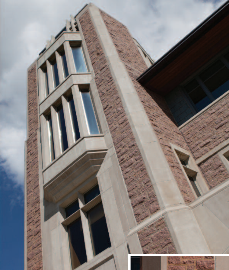
MISSOURI RED GRANITE AND INDIANA LIMESTONE AT PLAY IN A DETAIL FROM THE BAUER HALL SIDE OF THE NEWEST BUILDING IN THE OLIN SCHOOL OF BUSINESS. ACCORDING TO JOHN SMITH, PRESIDENT OF JOHN J. SMITH MASONRY, EACH PIECE OF RED MISSOURI GRANITE ON THIS BUILDING IS HAND CRAFTED IN THE MASON CONTRACTOR'S WORKSHOP.
