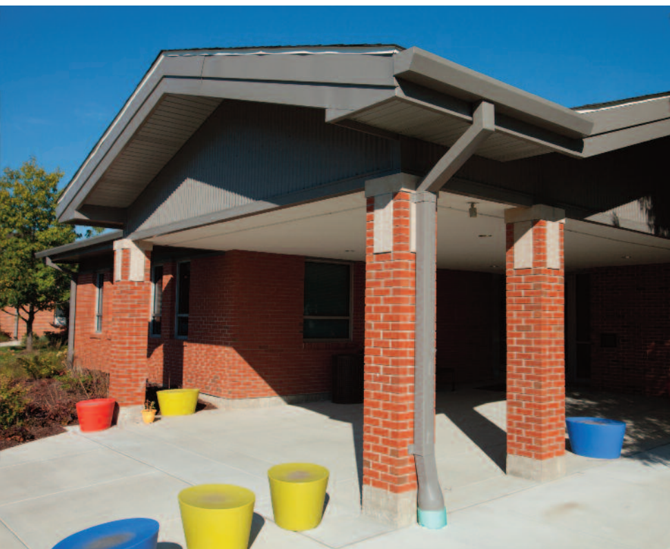
THIS FRONT ADDITION TO MABEE HALL ADDED A NURSING STATION AND AN OFFICE BULLPEN TO THE BUILDING. THE ADDITION OF THE BRICK PIERS AND VESTIBULE WAS DESIGNED TO PROVIDE THE RESIDENTS WITH A WELCOMING FRONT PORCH.
