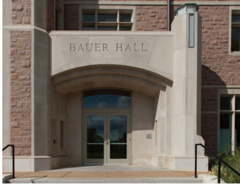
INDIANA LIMESTONE DEFINES THE VARIOUS ENTRANCES TO THE NEW ACADEMIC HALL.
