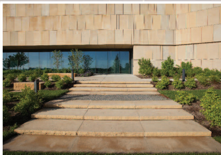
MOKETA LIMESTONE IS HARDER THAN NATIVE MISSOURI LIMESTONE, MAKING IT PERFECT FOR THE APPLICATION IN THIS RAIN SCREEN.
