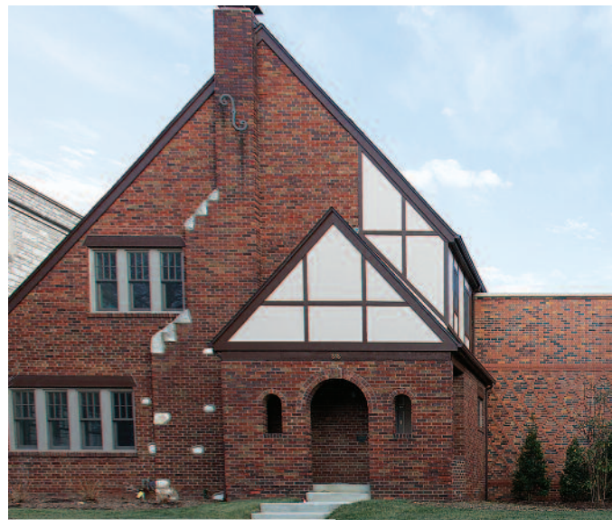
THE DIAMOND PATTERN ON THE NEW BRICK WALL LINKING THE TWO HOUSES OF THE NEW STUDENT CENTER MATCHES AN ORIGINAL PATTERN ON ONE BUILDING'S FAÇADE.
