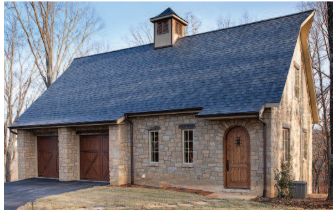
A MULTI-LEVEL "BANK BARN" BUILT INTO A HILLSIDE COMPLEMENTS THE OLD WORLD FEEL OF THE HOUSE BY USING THE SAME COMBINATION OF EW GOLD LIMESTONE BLOCK, BRUSHED MORTAR AND ANTIQUE TIMBER THAT IS USED ON THE HOUSE.
