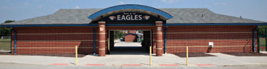
THE RESTROOMS AND CONCESSION STANDS AT THE SCHOOL’S FOOTBALL FIELD ARE CONSISTENT IN DESIGN AND CONSTRUCTION TO THE SCHOOL.
