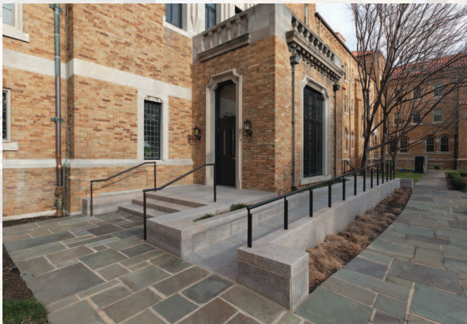
A NEW ADA COMPLIANT ENTRANCE IN THE BUILDING'S COURTYARD IS MADE OF STRUCTURAL MASONRY ACCENTED WITH GRANITE WALLS.
