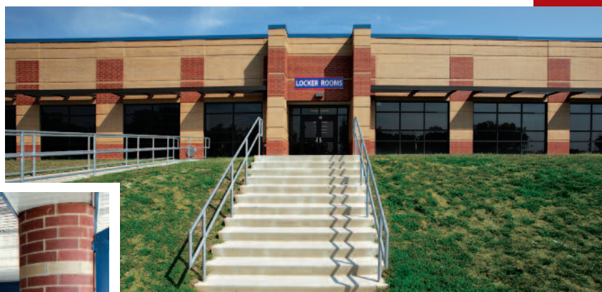
ABOVE: THE SOUTHERN FACE OF THE SCHOOL OFFERS ANOTHER VIEW OF THE CREATIVE USE OF MULTI-COLORED BRICK. HERE THE COLUMNS OF THE WINDOW BAYS EXTEND IN A DECORATIVE PATTERN BY USING A COLOR CHANGE TO CARRY THE DESIGN UP TO THE ROOF LINE.
