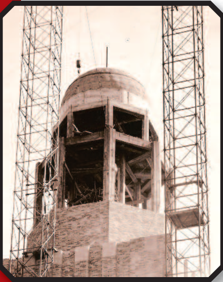
BELOW: INSTALLATION OF THE DISTINCTIVE BELL TOWER, 1930.
