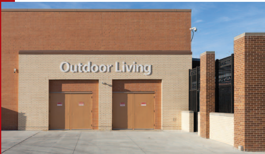
ABOVE: BRICK VENEER OVER LOAD BEARING MASONRY ACCOUNTS FOR HALF THE WALLS AT THE NEW FLORISSANT WAL-MART. MASONS FROM BRICKLAYERS' UNION LOCAL #1 OF MISSOURI AND EASTERN MISSOURI LABORERS' DISTRICT COUNCIL RAN 150 FEET OF WALL AT A TIME.
