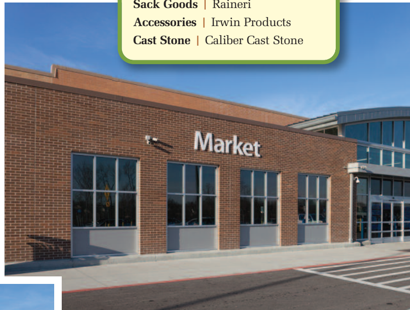
ABOVE: BRICK VENEER OVER LOAD BEARING MASONRY ACCOUNTS FOR HALF THE WALLS AT THE NEW FLORISSANT WAL-MART. MASONS FROM BRICKLAYERS' UNION LOCAL #1 OF MISSOURI AND EASTERN MISSOURI LABORERS' DISTRICT COUNCIL RAN 150 FEET OF WALL AT A TIME.
