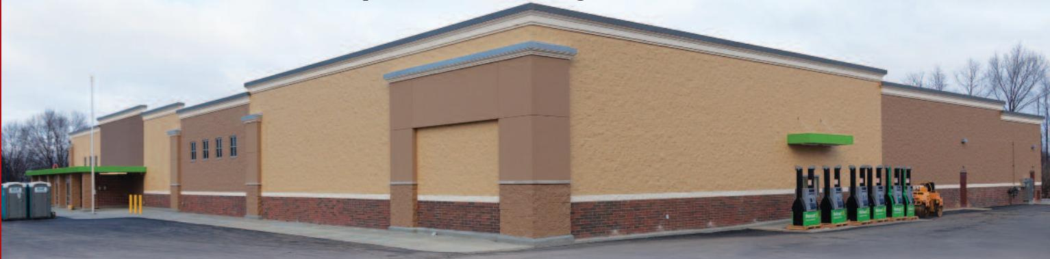
THE NEW WAL-MART NEIGHBORHOOD MARKET AT MID-RIVERS MALL DRIVE IN ST. PETERS FEATURES SINGLE WYTHE LOAD BEARING MASONRY WALLS.
