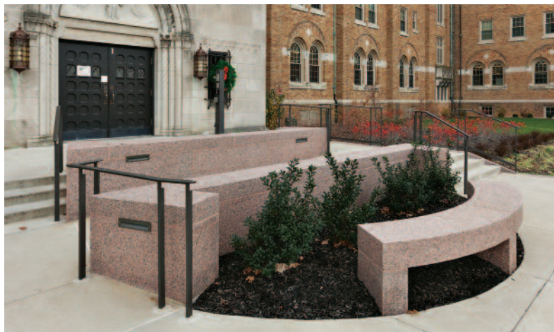
GRANITE WALLS AND A GRANITE BENCH GIVE THIS HANDICAP ACCESSIBLE ENTRANCE TO THE UNDERGRADUATE BUILDING AN ADDITIONAL USE AS A COMMON SPACE.
