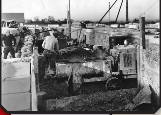
ABOVE: MIXING MORTAR IN 1929. NOTE THE LIME PITS.
