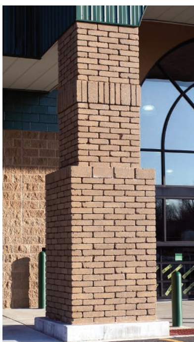
BELOW: BRICK PIERS AT THE ENTRY REINFORCE AN IMAGE OF STRENGTH AND STABILITY.
