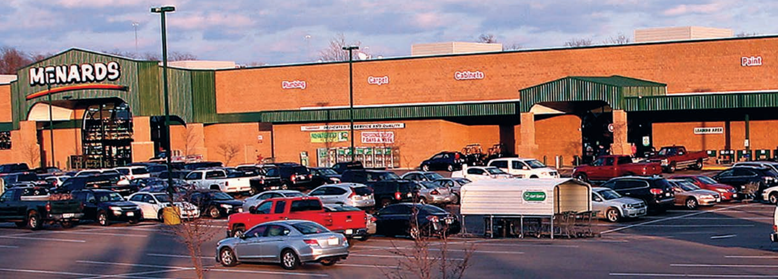
THE NEW MENARDS SUPERSTORE IN ST. PETERS WRAPS CMU AROUND THE BUILDING ENVELOPE, A MIX OF STRENGTH AND BEAUTY.
