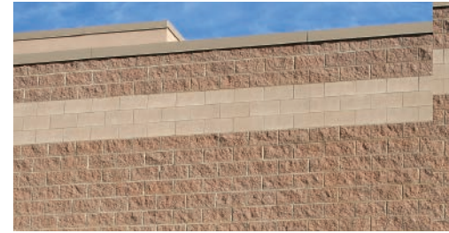
BLOCK COURSES OF DIFFERING TEXTURES ADD VISUAL INTEREST WHILE EFFECTIVELY BREAKING DOWN THE MASS OF THE BUILDING ENVELOPE.
