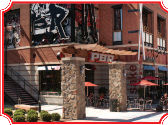
CULTURED STONE ON THE ENTRY COLUMNS (BELOW) AND OUTSIDE OF PBR, A COWBOY-THEMED BAR, WAS INSTALLED BY JDS MASONRY.
