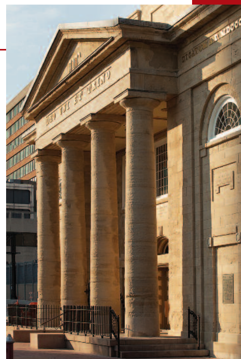
ABOVE: AN OLD PLASTER LAYER COVERING THE BUILDING’S DORIC COLUMNS WAS REMOVED, THEN THE COLUMNS WERE CLEANED AND REDRESSED. MASONRY PLASTER WAS USED ON THE BASE OF THE COLUMNS TO MIMIC THE MARBLING LOOK ON THE COLUMNS. BELOW: NEW MEDALLIONS WERE FABRICATED. EVERY EFFORT WAS MADE TO BLEND THE NEW STONE WITH THE ORIGINAL.
