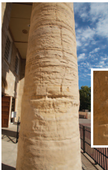
A DUTCHMAN REPAIR ON ONE OF THE COLUMNS. THE ORIGINAL LIME MORTAR WAS REFORMULATED AND USED TO REPAIR ALL JOINTS ON THE COLUMNS AND FAÇADE.
