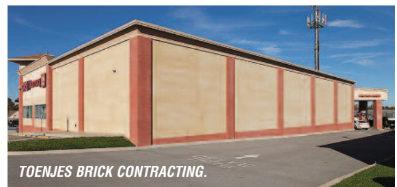
TOENJES BRICK CONTRACTING. A PORTION OF THIS SHOPPING PLAZA WAS DEMOLISHED SO A NEW PHARMACY WITH A DRIVE THRU COULD BE BUILT.
