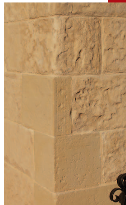
DETAIL OF NEW STONE ON A CORNER OF THE OLD CATHEDRAL.
