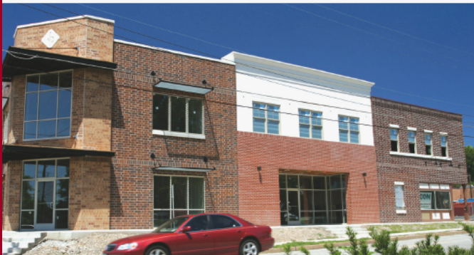
THANKS TO MAPLEWOOD'S RECENTLY-ENACTED MASONRY ORDINANCE, JAMES PLACE IN MAPLEWOOD IS A NEW FOUR-SIDED MASONRY DEVELOPMENT AT SUTTON AND JAMES AVENUES. THE 10,000-SF. PROPERTY WILL CONSIST OF RETAIL ON THE FIRST FLOOR AND MEDICAL ON THE SECOND.
